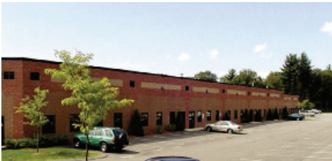
155 Northboro Road - Southborough, MA
